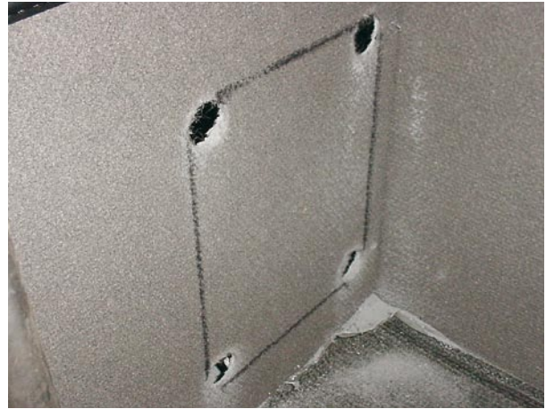
Figure 8 - Location for cutting return air vent
